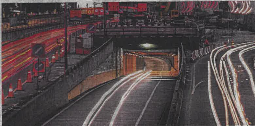
The Stormwater Management And Road Tunnel has been featured alongside other prominent tunnels in top documentary channels. PIC BY AIZUDDIN SAAD
