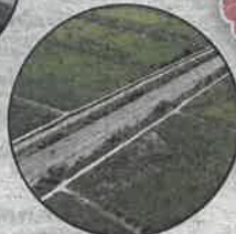
BUTTERWORTH-KULIM EXPRESSWAY (BKE) Length: 17 km
