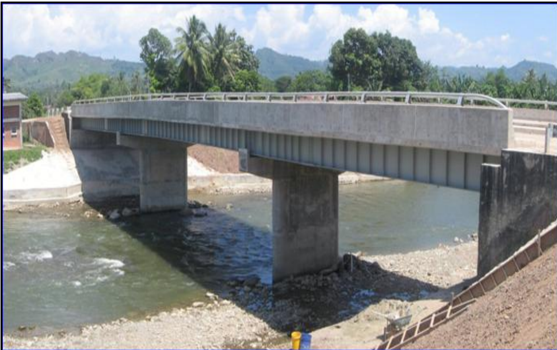
Sub-Pakej 5 - Gasabun Bridge, Keningau
