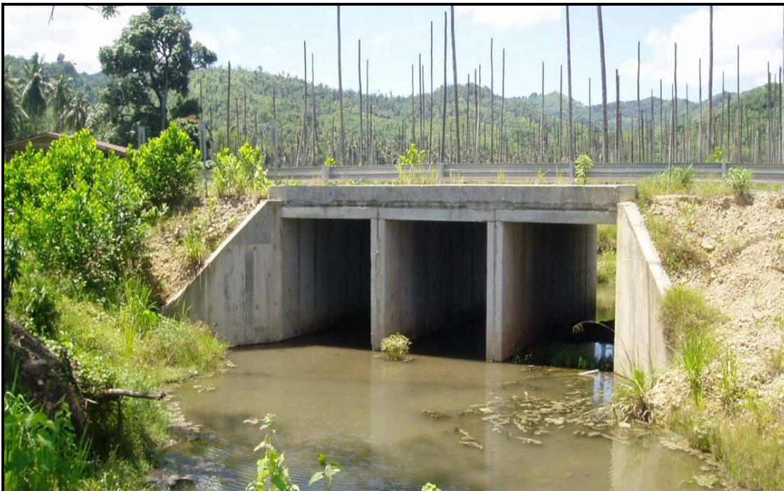
Sub-Pakej 4 - Box Culvert at Sg. Gailun, Pitas
