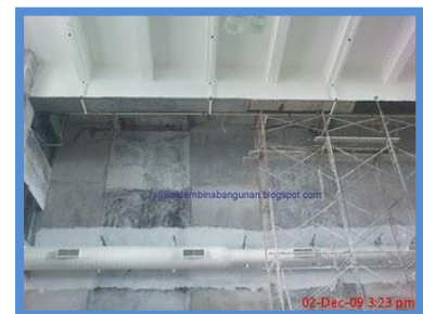
Pemasangan air-cond duct
